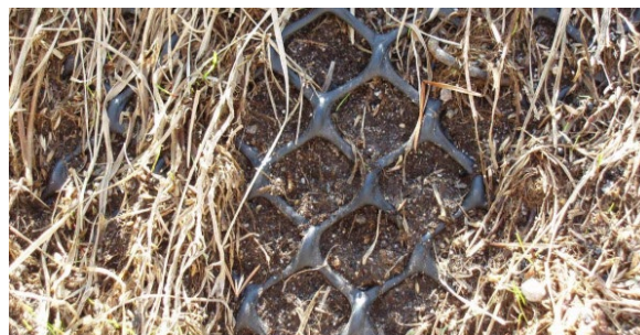
Permanent plastic lattice
